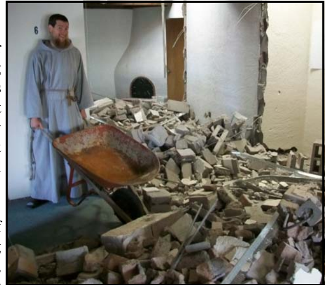
Br. Gerard working on interior demolition
